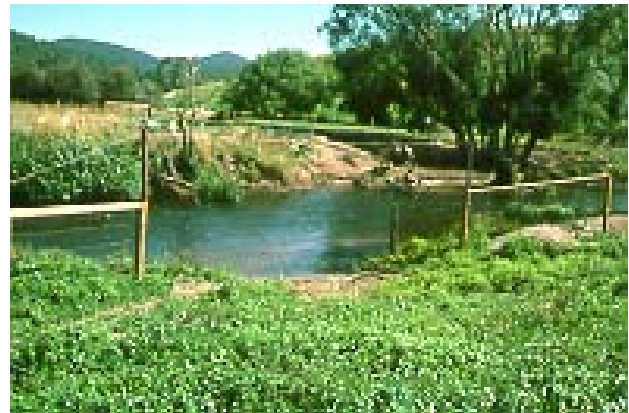
A two-wire electric fence, with livestock access 'chutes' (gravel ramps), protects the stream environment and livestock from drowning. An even better option might be total exclusion and provision of water in troughs.
