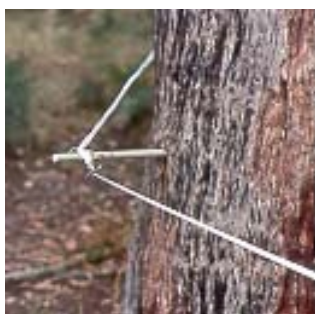
A tree has been used as a corner post for an electric fence erected to protect native vegetation. A steel pin avoids the need to circle the tree with wire which may eventually kill it or create a hazard if the tree is ever sawn.
