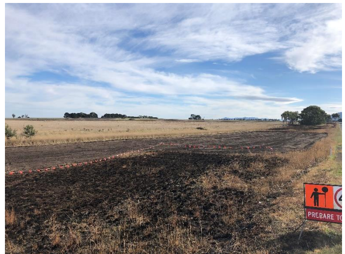
Soil scalping on Penshurst-Dunkeld Road
